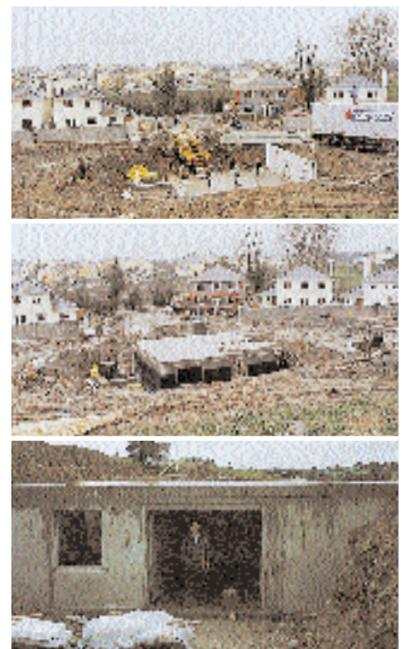
▲ Bob Noonan's basement extends under the whole of his home in County Clare. He chose the Swedish ThermoneX system, which uses highly insulated precast concrete panels.
