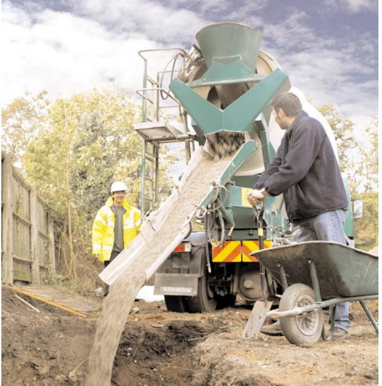
(the general choices being 450mm and 600mm wide). Using a 450mm wide bucket is going to reduce the amount of readymix used by a quarter (as well as reducing excavation costs) but it is not to be recommended to inexperienced builders. Cavity walls – generally now 300mm wide – sit uncomfortably on such a narrow trench; single skin brick masonry (as used in the garage) is obviously less of a problem but the key factor in all this is accurate setting out of trenches.
