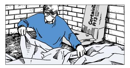
Cover the ground with the polyethylene sheeting, overlapping joints by 12" or more. Then use the rocks or boards to hold the material in place. This will prevent ground moisture from entering the space, rising to the flooring above and causing mold or wood rot.
