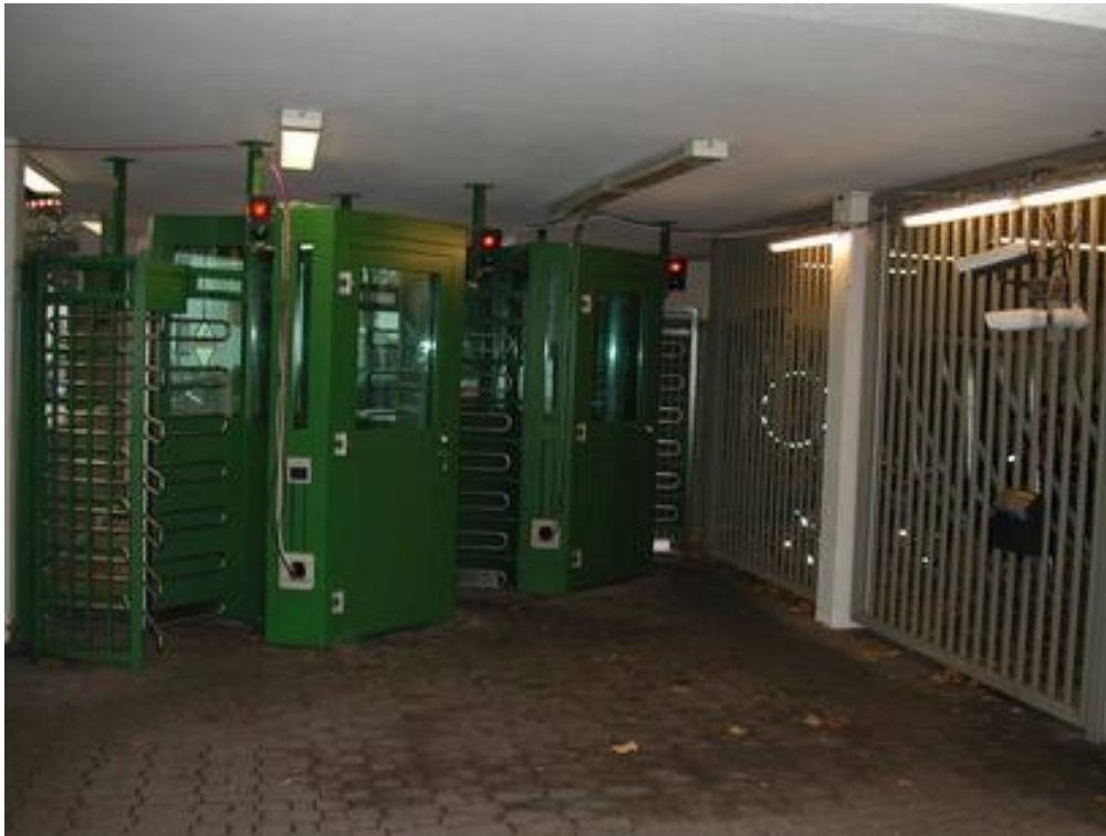
Figure 117: overview of the system test installation
