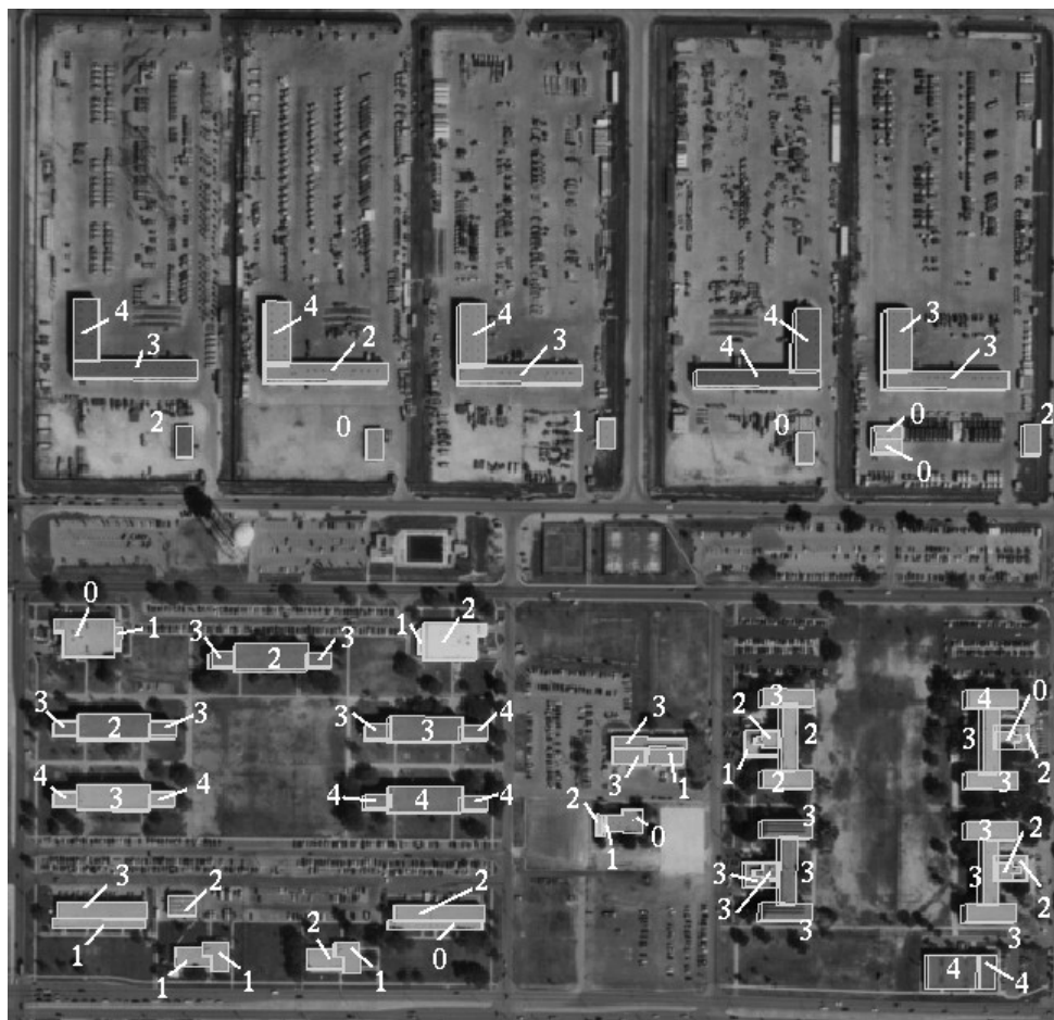
Figure 15: The ground truth model projected into image 713. The number of times each roof facet polygon was detected over the four different views is overlaid to depict an overall 2D detection rate of 89% for batch-mode processing at 0.7 sensitivity setting. Higher detection rates are possible but at the expense of more false-positives. The sensitive setting 0.7 was chosen as a reasonable setting that detects a large number of roof facets, while attenuating the number of incorrect detections.
