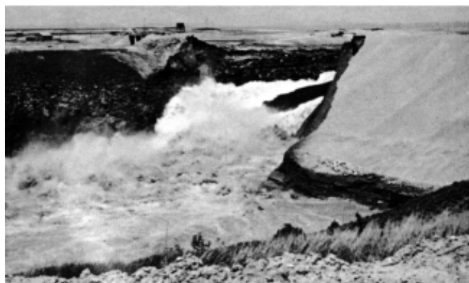
Figure 22. Sequence of photos taken during the failure of the 90 m high Teton Dam. These three photos were taken at 11:20 a.m., 11:50 a.m., and the early afternoon of June 5, 1976 (from Chadwick, 1976). Over a period of hours, piping through joints in the key trench area eroded the core material from within, undermining the north side of the dam.
