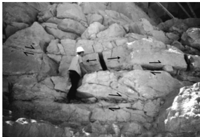
Figure 12. Open vertical to steeply-dipping cooling fractures offset by horizontal shear zones in the north key trench Zone 2. Both sets of open joints allowed piping of water from the reservoir, which eroded the core of the dam and caused its failure. Arrows indicate relative motion along shear zones, see Figure 14.
