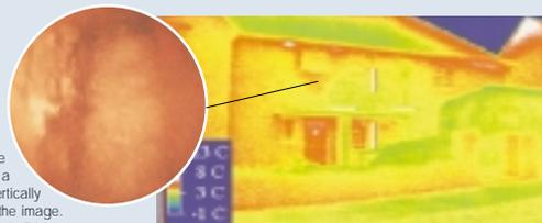
This boroscope image shows the mineral fibre as a band running vertically in the centre of the image. The mineral fibre is 500mm away. This is a large void.
