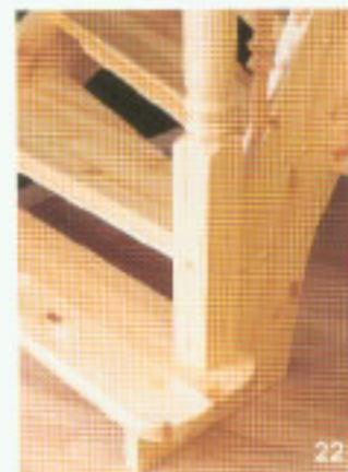
Open bullnosed tread curved on one side. The opposite side is placed against the wall.
