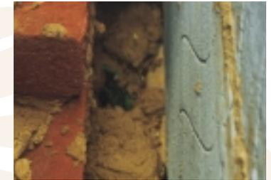
This image shows the accumulation of mortar on the top surface of mineral fibre full fill batts amongst other elements of poor workmanship.
