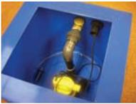
The concept of the drained cavity system is to collect and manage any moisture which breaches the integrity of the structure by channeling, collecting, and discharging such free water via a suitable evacuation point."
