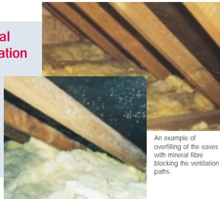
An example of overfilling of the eaves with mineral fibre blocking the ventilation paths.
