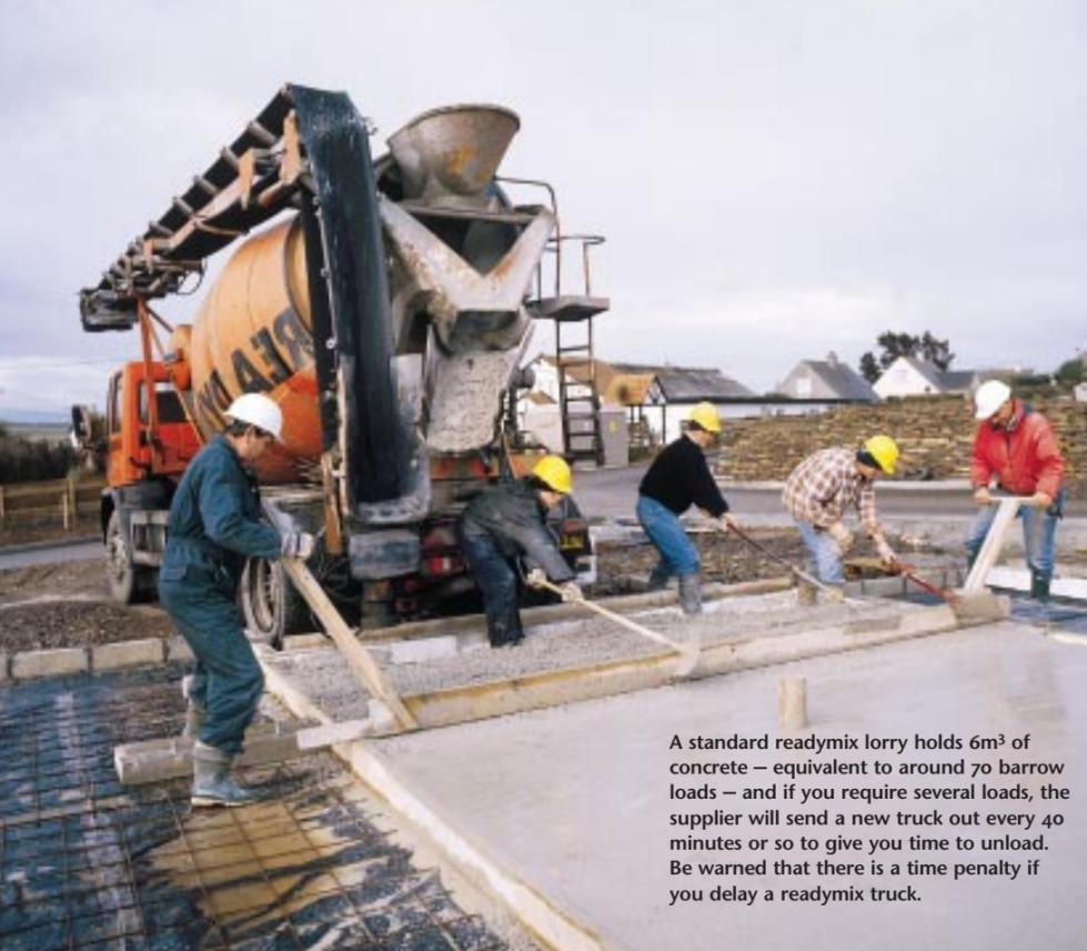
A standard readymix lorry holds 6m<sup>3</sup> of concrete – equivalent to around 70 barrow loads – and if you require several loads, the supplier will send a new truck out every 40 minutes or so to give you time to unload. Be warned that there is a time penalty if you delay a readymix truck.
