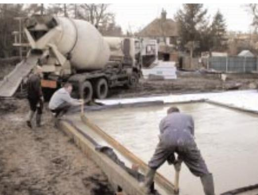
▲ Most new homes have a poured oversite slab, comprising of compressed hardcore, a dpm layer, insulation and 100mm of readymix, tamped down to remove air and leave a smooth, level surface.
