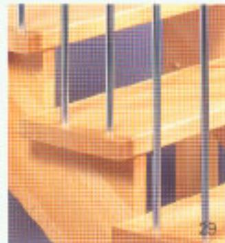
With stepped treads the spindles are drilled into the tread.
