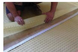
The %R.H. Levels are isolated in the air gap, and controlled. Delta membranes can be used in new build, remedial or refurbishment projects for floors, and walls.
