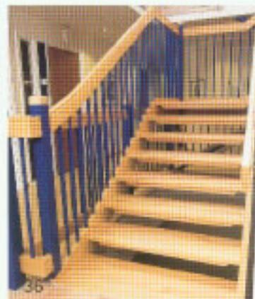
36 Stair with zero step, e.g. floor and first tread are at same level.
