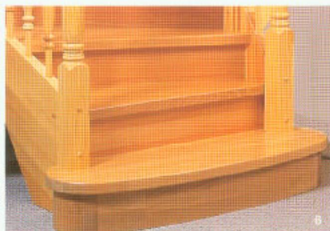
Treads/risers in solid beech varnished, strings in pine. Bullnosed tread with curved front edge.
