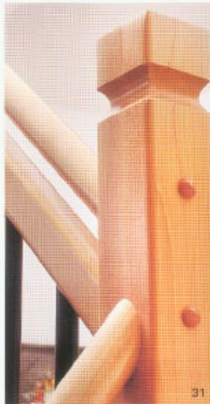
Raking balustrade with a "floating handrail" which goes free from the spindles. Same design can be made against the string, the spindles are then drilled into a "floating piece of wood" which is distanced from the string. This is called "floating balustrade".
