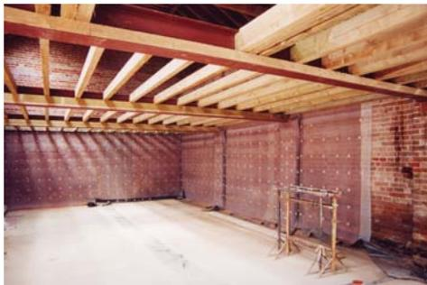
dabs and a skim coat of Thistle Multi finish. The stable block was over boarded with thermal insulation Board.
