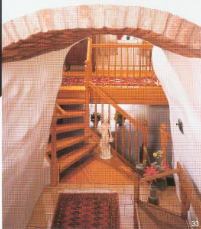
33 Half-turned stair with three-cornered integrated landing. Whole stair in antique-stained solid oak. Spindles no. 3, newel post type G.
