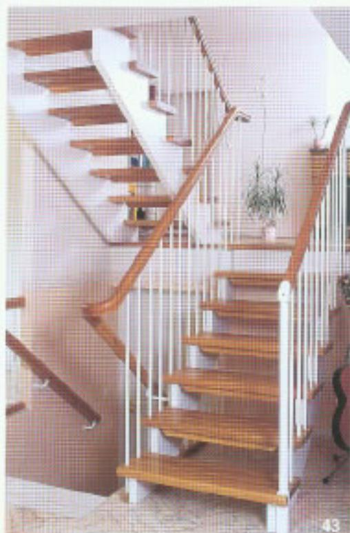
Straight flight of stairs with stepped treads in solid oak and white-painted strings. White spindles no. 14.
