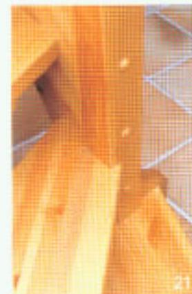
To mark the stair corners, stronger posts which are joined to the treads and strings are used.
