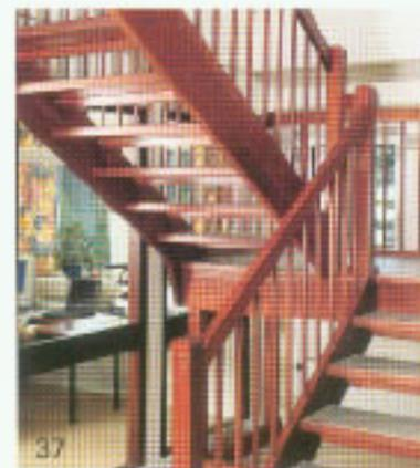
37 Connection of stair flight to landing. Strings integrated with landing sides.
