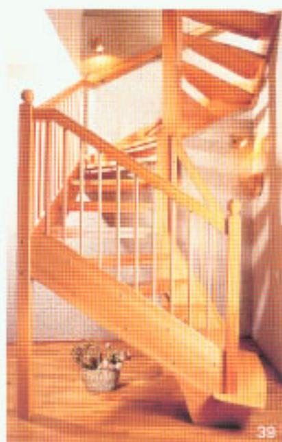
Square-turned stair in varnished beech. Bullnosed tread with curved front edge. Spindle no. 4, post type C.
