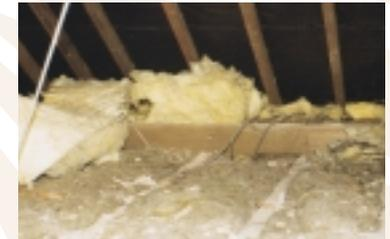
This image shows the additional layer of mineral fibre missing over a substantial portion of the attic.
