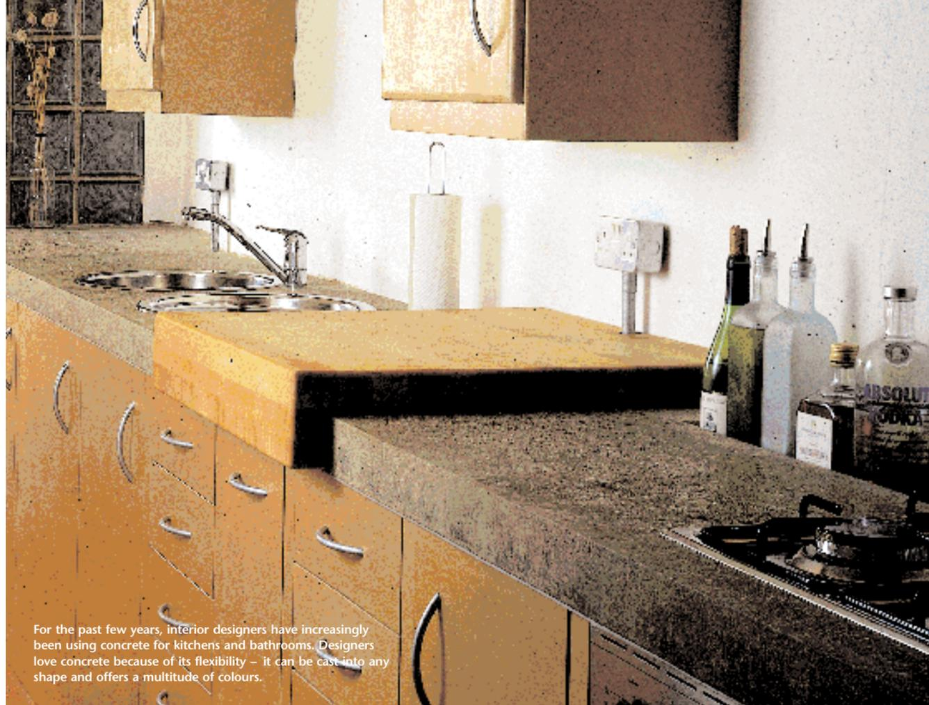
For the past few years, interior designers have increasingly been using concrete for kitchens and bathrooms. Designers love concrete because of its flexibility – it can be cast into any shape and offers a multitude of colours.
