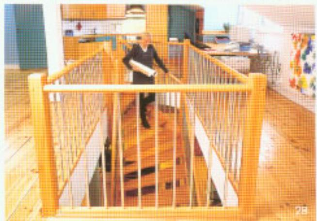
Horizontal balustrade round stairwell. Handrail no. 5 in varnished beech and spindles no. 14 (polished metal). Newel post type D.
