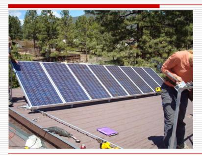
Typical roof top installation uses a rack mounting system, panels set in arrays or "strings" (multiple panels) and conduit for interconnection of panels. Shown here are Sharp 170s. A cell or module is a single silicon unit and generators 0.5 volts.
