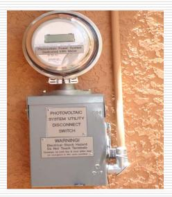
Note: More warning labels are required adjacent to the inverter and DC disconnect at the roof location. Once APS or the utility company authorizes the connection to the grid, a secondary digital meter with remote reading capability will be added to the service panel. During a light usage day and with full sunlight, the service panel meter will run "backwards".
