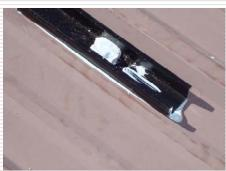
This "standoffs" or spacers of this Pro-Solar system is attached using 5/8" diameter, 3" long lag bolts through the metal roofing, ½" OSB and penetrating the 2-1/8" wide TJI top chord webs. The holes are pre-marked and drilled. Henry's 9000 gutter and flashing sealant is used to prevent roof leakage.
