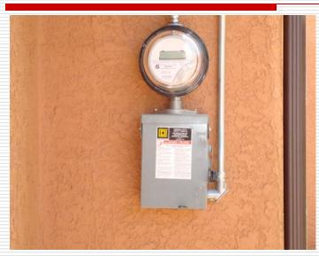
A digital AC "power" production meter is installed after the lock out junction box for the system. The Utility Company (APS) wants this lock out accessible without going into a fenced backyard. The meter must be read once a year and the information sent to the Utility Company within 15 days.
