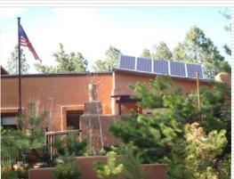
From the street side, this roof top solar panel generating system (5.61 Kwh) awaits the City inspection and "green tag". Once that it completed, APS is scheduled to replace the service panel meter with a bi-direction digital meter and approve the installation for operation. Then during the peak months, the owner hopes to run the meter backwards as it generates more than used.
