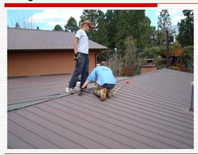
The layout crew will measure the surface area of the roof and must check the exact location of the roof framing members beneath. Since the panels add a tributary load of between 3-5 psf, this extra dead load is minimal and should not require a structural engineer. However, the rack system requires that the anchors are embedded into the roof framing, not just the sheathing.
