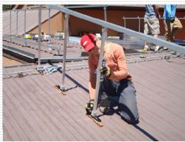
The installer works to keep the legs and rails plumb. Care is given during the "setup" stage to prevent having to disassemble or make major adjustments once the panels are installed. This system has a total of 33 Sharp 170 watt panels or a maximum production of 5.61 Kwh. The layout and rack installation took 2-1/2 days to complete (prior to installing any panels).
