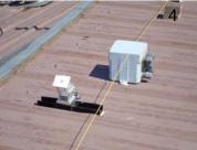
Photos: #1, wire spool racks with 10 gauge wiring and color coded make the pulling of wires easier. #2, the DC switch with grounding and lug terminals are used to connect the arrays to the inverter (this is a Sun Boy 6000). #3, junction boxes and conductors are elevated above the roof deck to prevent damming of leaves and debris during rain and snow storms. #4 The conduit is held up from the decking with artificial decking blocks (predrilled) and caulking; string line keeps system aligned.
