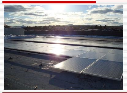
The racking system for this installation is laid flat on the built up roofing system. Care must be taken to interconnect the panels before they are lowered and connected. Obviously, maintenance to an interior panel is more complex.
