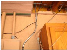
Since this panel is exterior to the house (open to the environment), the panel needs to be connected through the bottom of the existing service panel. The bare copper wire is connected to the service panel grounding lug and uses the existing UFER to complete the ground.
