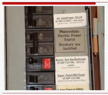
Feed breaker may not exceed 20% of the panel service size. This case, the house service was 200 amps, this limits the breaker to 40 amps; max. output for this system is 25 amps. During final inspection, it was determined that the wiring size (10 gauge) needed to be a double pole 30 amp fuse or increase the wire size to #8s for the 40 amp breaker. Breaker was changed.
