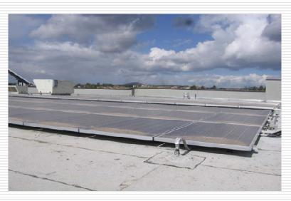
The electrical boxes (at ends of panel arrays) and conduit with conductors for the connections to the inverter bank(s) are snaked through a roof mounted and protected conduit (shown in the foreground).
