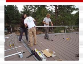
Although installation could be done by one individual, a multi-crew installation makes holding the rails to the vertical supports much easier. These rails are aluminum and easy to cut and hold in place.
