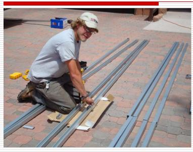
The alum. "C" channel shaped rails are connected together and must have a grounding bond between the rails. Charlie is securing a pre-drilled connector that will snuggly clamp two twenty foot sections together. A bonding scrap, using a lock washer straddles the two channels and is tightened down. The Weeb splicers are used as the grounding is not sufficient with just the ProSolar splice kit.
