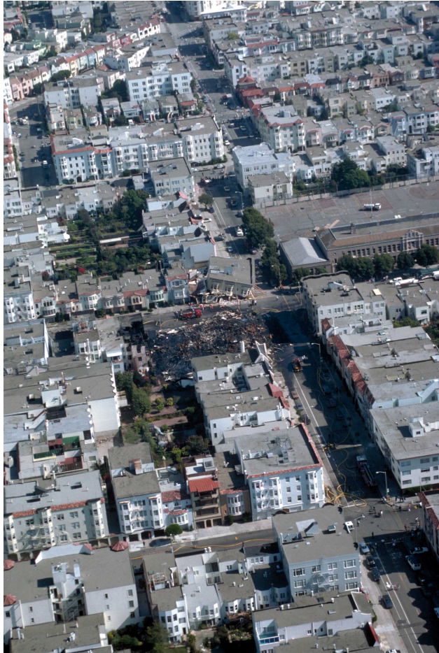
4. Aerial view of collapsed buildings and burned-out section at Beach and Divisadero Streets, Marina District . [C.E. Meyer, U.S. Geological Survey]
