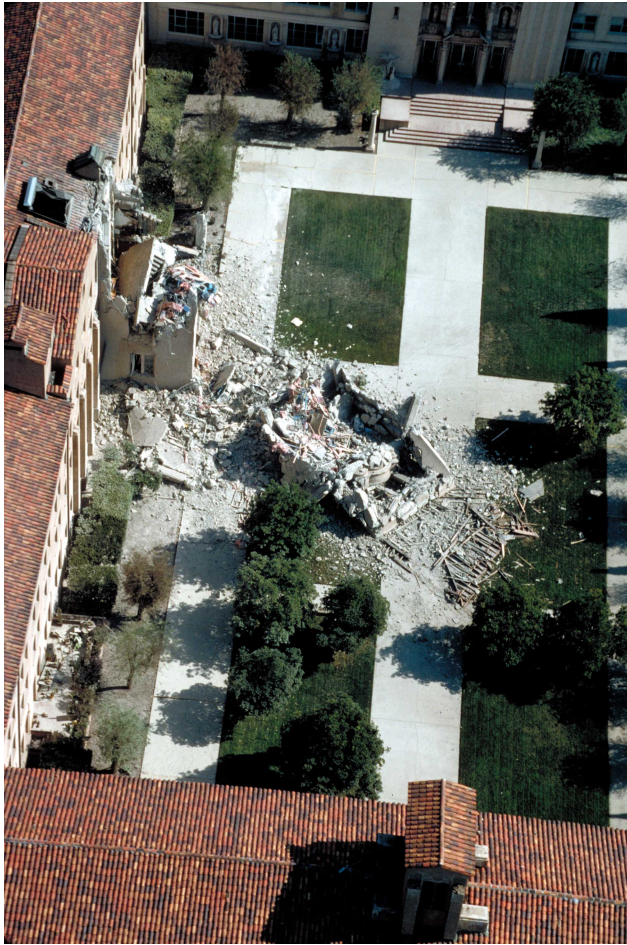
43. Aerial view of collapsed five-story tower, St. Joseph's Seminary. [H.G. Wilshire, U.S. Geological Survey]
