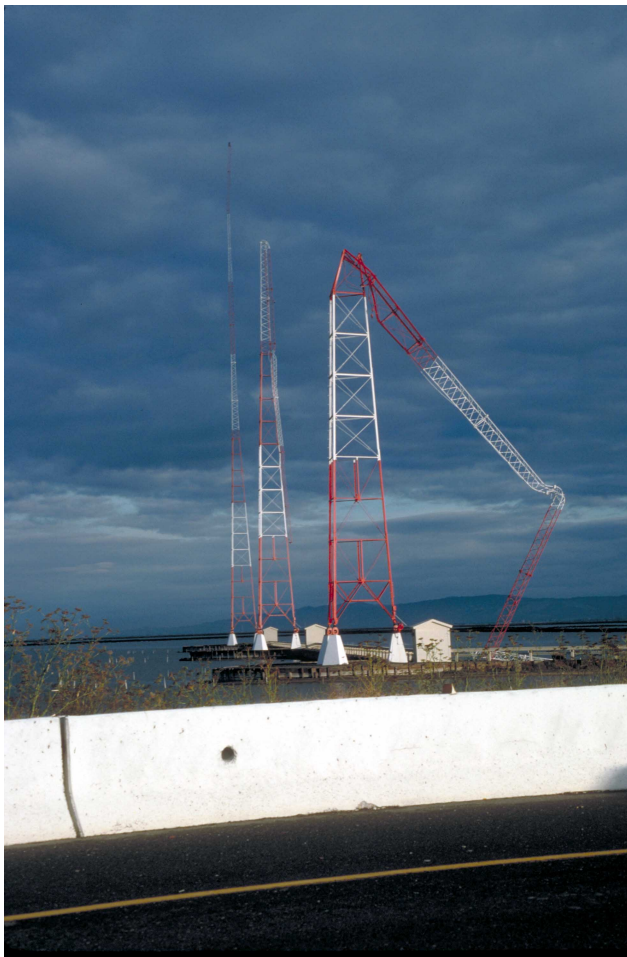
37. KGO radio transmission towers, built on bay mud in a salt-evaporation pond used by the Leslie Salt Company. Note progressively less damage to towers away from viewer. [H.G. Wilshire, U.S. Geological Survey]
