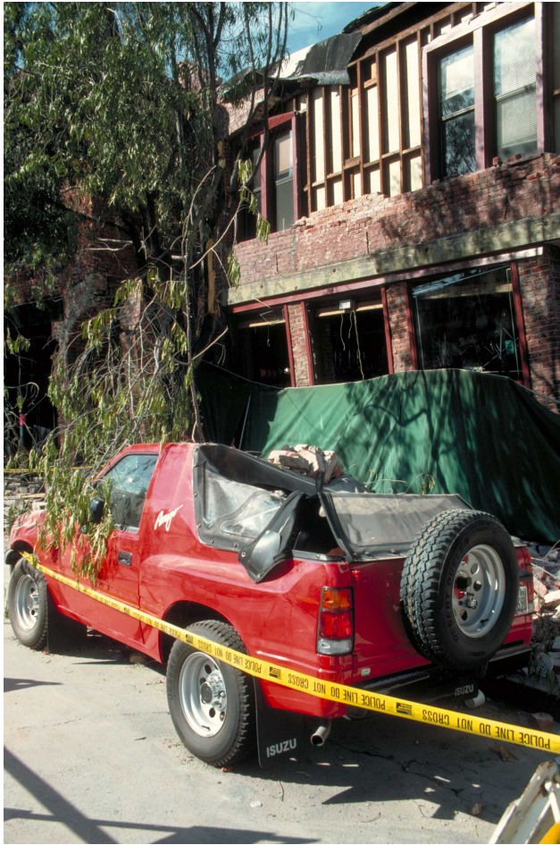
51. Vehicle crushed by collapse of unreinforced-brick masonry. [C.E. Meyer, U.S. Geological Survey]
