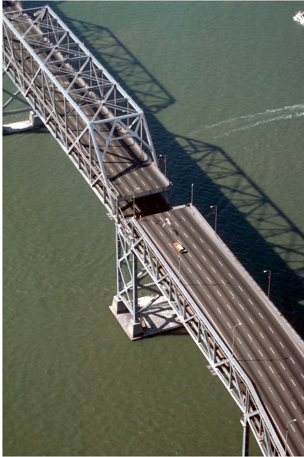
16. Aerial view of the collapsed section of the San Francisco-Oakland Bay Bridge. View westward. [C.E. Meyer, U.S. Geological Survey]
