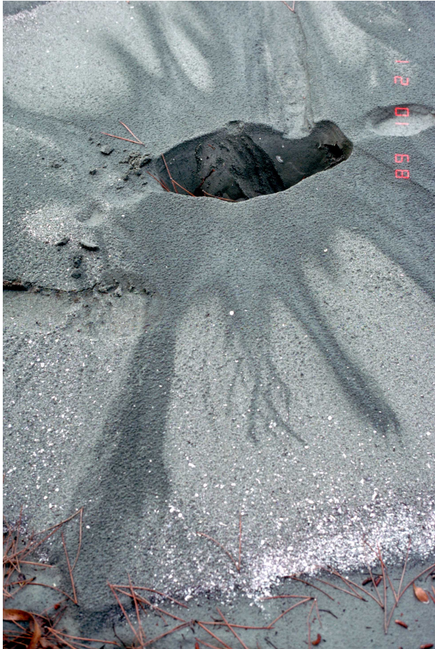
17. “Sand boil” or sand volcano measuring 2 m (6.6 ft) in length erupted in median of Interstate Highway 80 west of the Bay Bridge toll plaza when ground shaking transformed loose water-saturated deposit of subsurface sand into a sand-water slurry (liquefaction). Vented sand contains-marine shell fragments. [J.C. Tinsley, U.S. Geological Survey]
