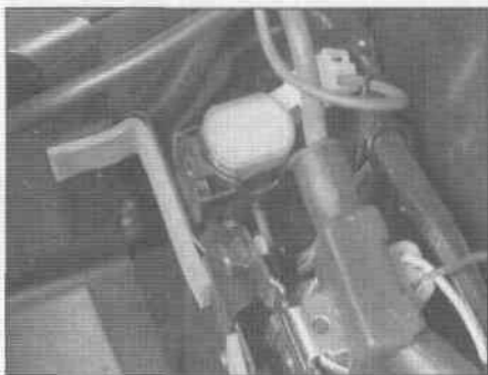
5.7a A circuit breaker is mounted under the seat (this is a Katana 1100/GSX1100F)..-
