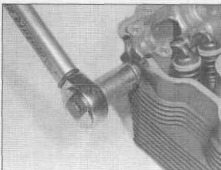
10.42 Install the rocker shaft plug with a new sealing washer
