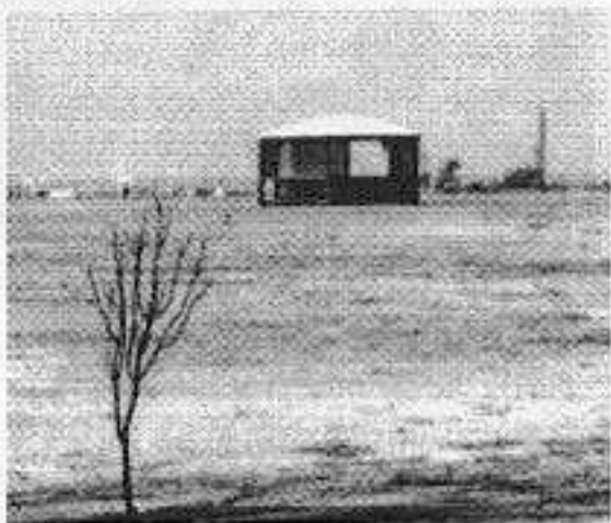
Structure built to test interference.
