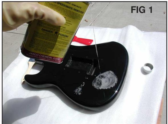
**IMPORTANT POINT:** If you can help it, avoid working in direct sunlight. The sun tends to dry the paint stripper before it can really do its work. A shaded area outside is preferable.
