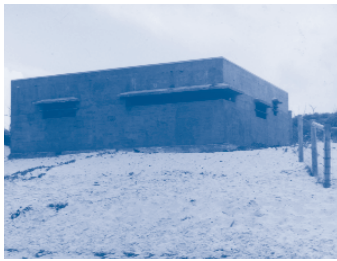
Photo 26.1 Shore station at Bribie Island, Queensland.
